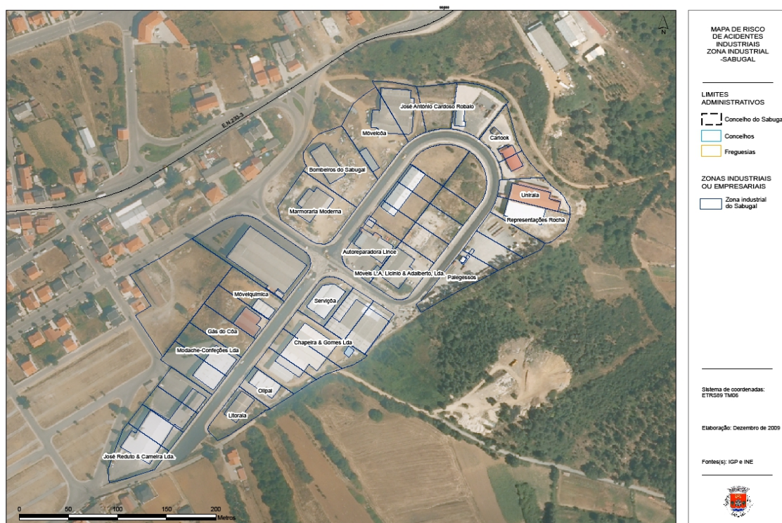
Figure 25 – Zona Industrial do Sabugal
